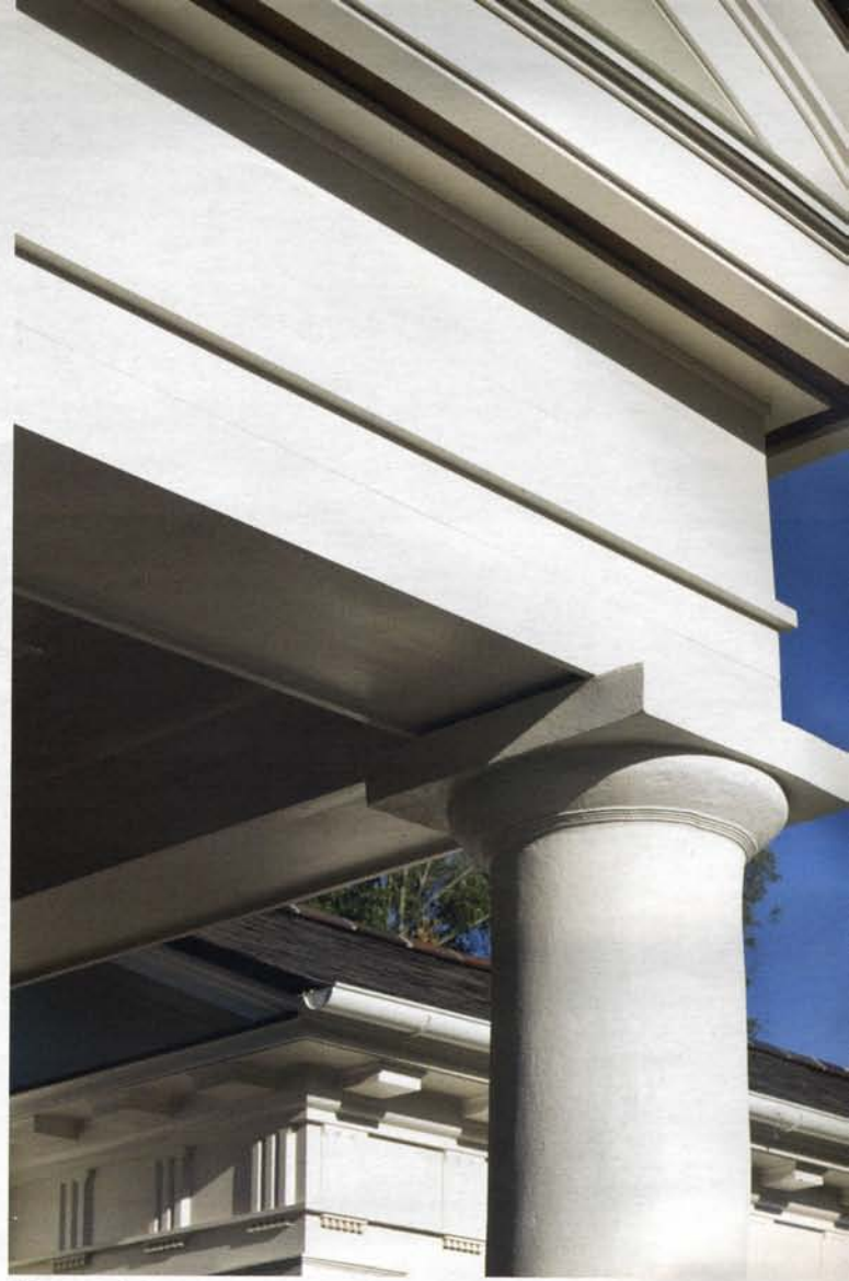
Above and above left: The pool house pediment is supported by masculine Greek Doric columns, which were constructed using traditional methods: stacked brick with a stucco overlay. The bricks used for the terrace are queen-sized Carolina handmade brick.
